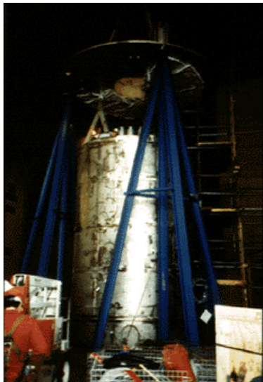
The heat exchanger prior to its installation inside the reactor vessel
