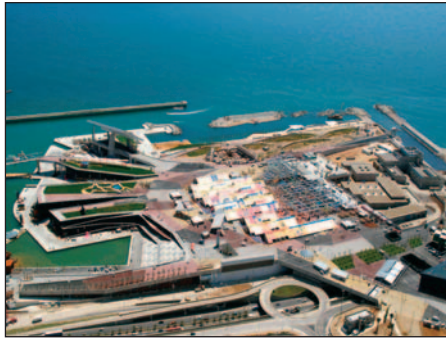
The new wastewater treatment plant
