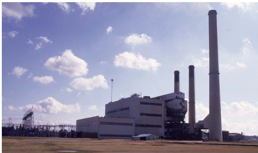
Alabama Power's Greene County Facility
